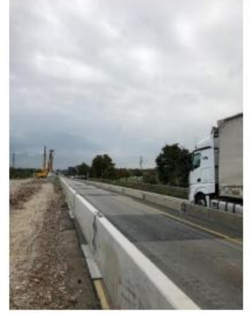
Figure 4-8 Example Shy Lines adjacent to Concrete Safety Barriers
