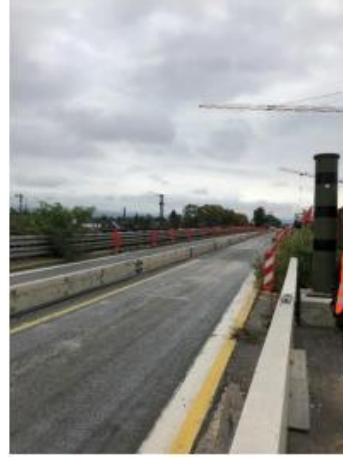
Figure 4-8 Example Shy Lines adjacent to Concrete Safety Barriers
