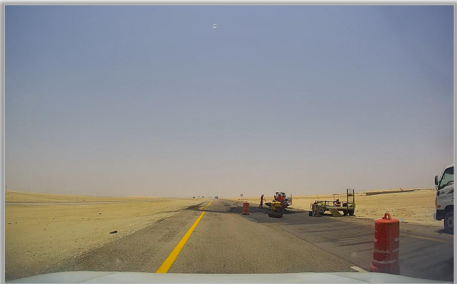
Equipment operating on the asphalt surface without sufficient protection
