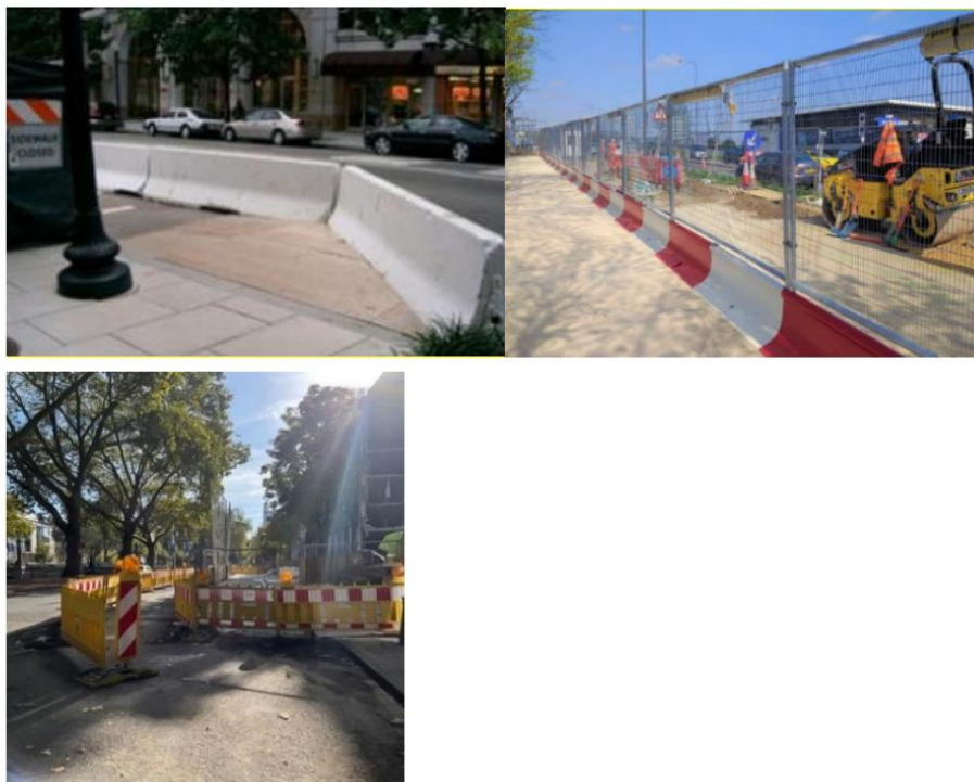
Figure 4-14 Pedestrian Protection around Construction Site incorporating Safety Barriers and Barricades (ARTBA, 2018; Source: Safe Site Facilities)
