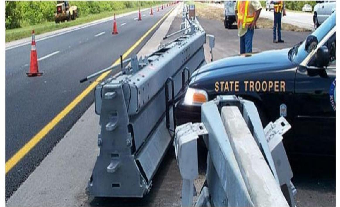
Figure 37. Median gate used for emergency vehicle access at a work zone.
