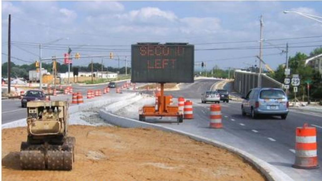
Figure 31. PCMS often need to be positioned in the roadway clear zone, where they pose a potential hazard to errant vehicles.
