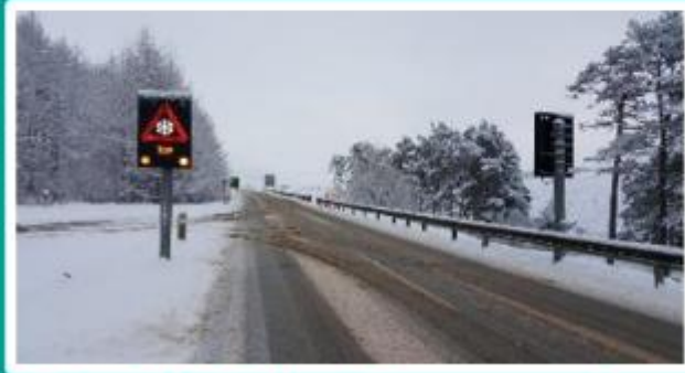
Road Weather Management: Ice/slippery road warning
