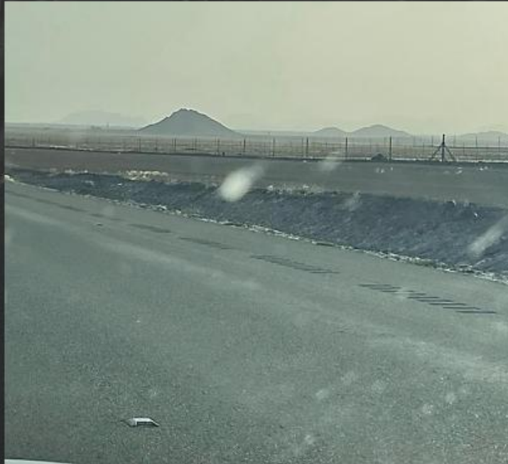
Drainage ditches, swales
