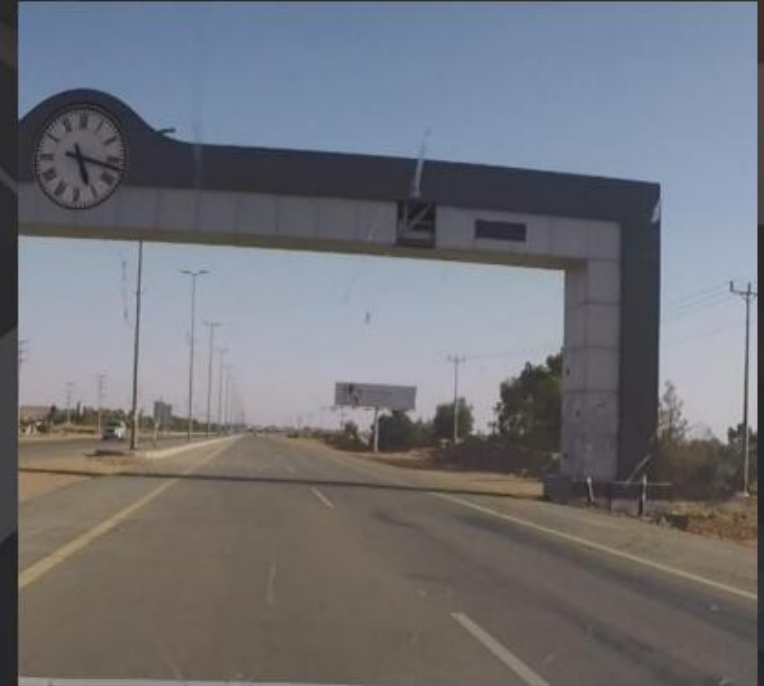
Buildings | Gateways Rock outcrops in cuttings
