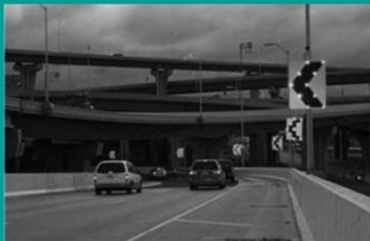
Sequential Dynamic Lighting Curve Warning Systems
